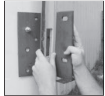
6. Level bracket and drill remaining 5 holes.
