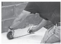
1. Locate the center points of the columns. Make sure the layout and slab are square. **NOTE:** The concrete slab needs to be a minimum of 5" thick. The concrete footing must be a minimum of 2'x2'x2' and needs to reflect the local building code requirements. Concrete must be a minimum of 2,000 psi.
