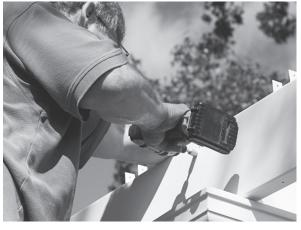
**15.** Install the rafter supports with the decorative rafter tails on the opposite side of the aluminum angle using 2.5" hex head stainless steel self-tapping screws. Set clutch on the drill so the screw is not stripped.
