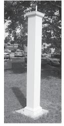
7. Position the column so that it is centered over the connector nut. If the column base is not installed, slide it over the top of the column and down the column to the bottom.
