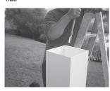
9. Lower the threaded rod into the column and engage the coupling nut on the bottom.
