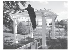
**19.** Set the clutch on the drill to ensure that the screw head does not dimple the top surface of the purlin. Continue across the top of the rafters until all purlins have been installed.
