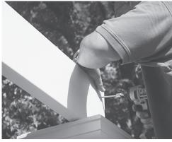
**14.** Install all the headers without decorative rafter tails to the outside of the aluminum angles on top of the columns using the 2.5" hex head stainless steel screws. Set the clutch on the drill so the screw is not stripped.
